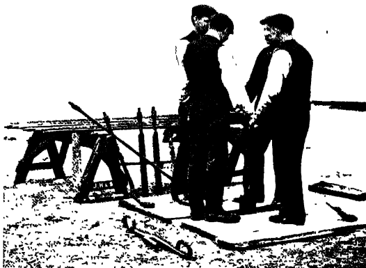
Fig. 13.—Hand Boring Plant.
